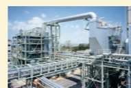
Biomass power plant (2005)
